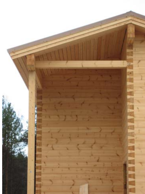
A VENEER-WEB PRT PILLAR-BEAM STRUCTURE WITH 300 MM OF INSULATION WAS USED IN A PILOT BUILDING IN OULU (RIGHT).
